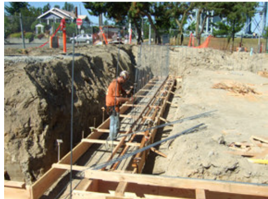
Setting rebar for the gym wall.
